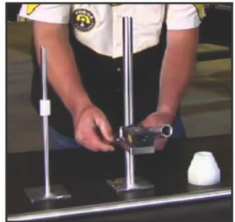
2. Install laser alignment tool.
